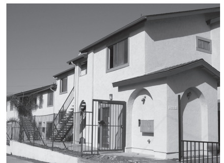
Second Chance 35th Street Apartments
